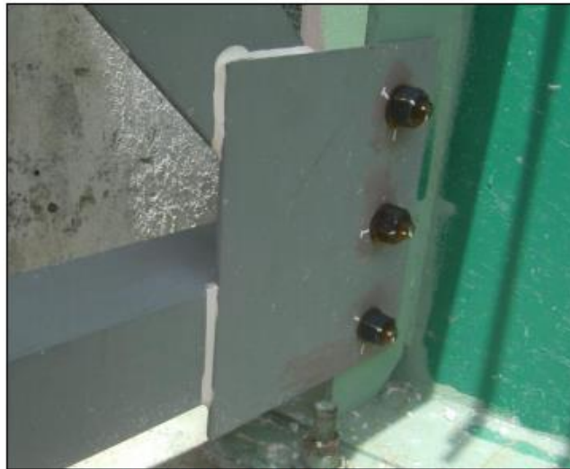
A Caulked Field Connection
