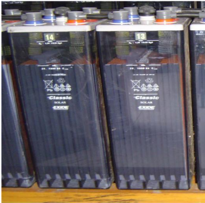
Gambar 35: Baterai Deep-Cycle
