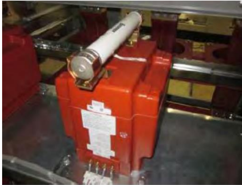
Gambar 4.26 Potential Transformer (PT)
