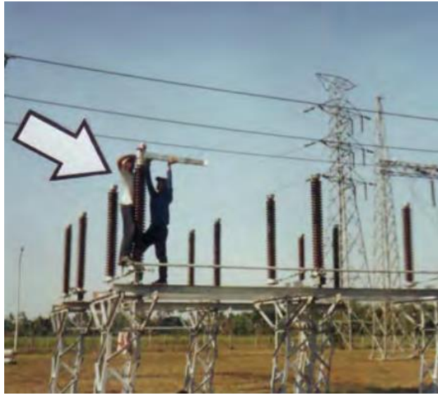
Gambar 4.23 Disconnecting Switch (DS)
