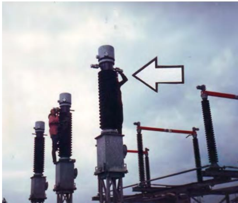
Gambar 4.25 Current Trasformer (CT)
