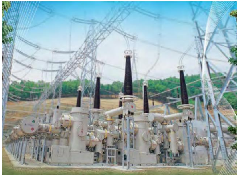
Gambar. 2.3 Gas Insulated Substation (GIS)
