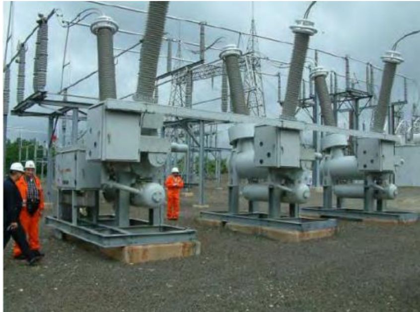
Gambar 4.22 Circuit Breaker (CB)
