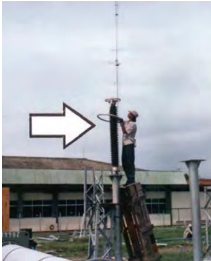
Gambar 4.24 Lightning Arrester (LA)
