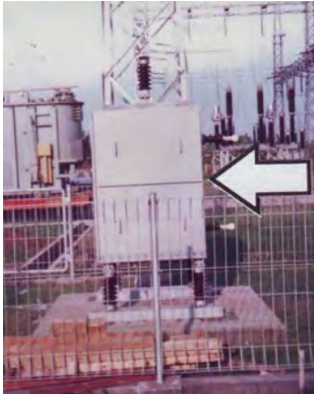
Gambar 4.21 Neutral grounding Resistance (NGR)
