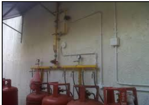
Gambar 33. Instalasi Pipa Gas Sistem Manifold
