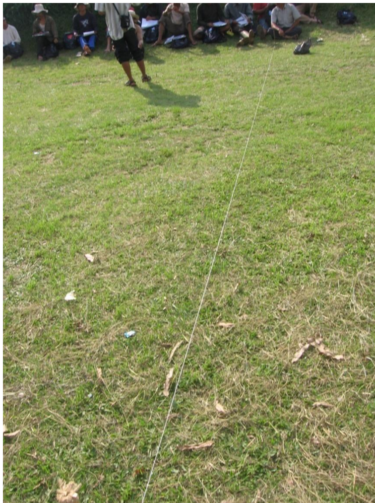
Gambar 184. Menarik garis as reaktor biogas
