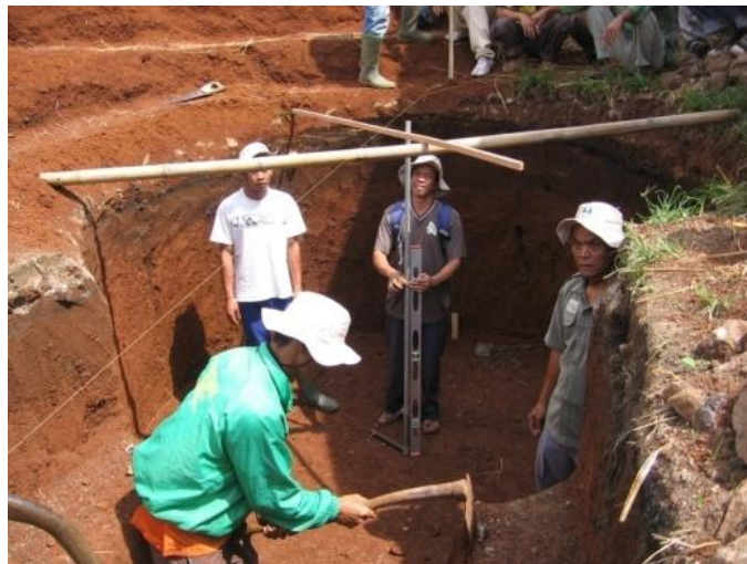
Gambar 44. Pemasangan tiang as
