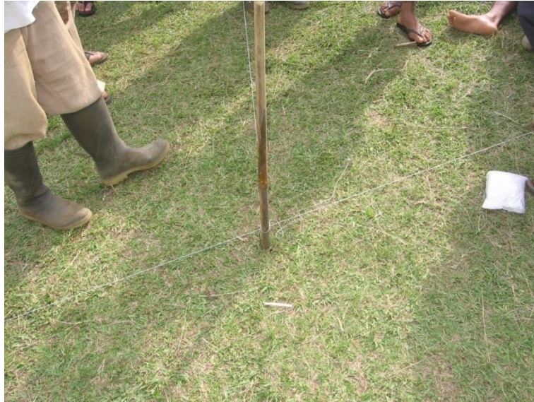
Gambar 185. Menentukan as tangki pencerna
