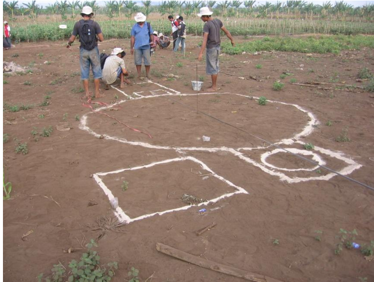
Gambar 191. Gambar lay out galian reaktor biogas
