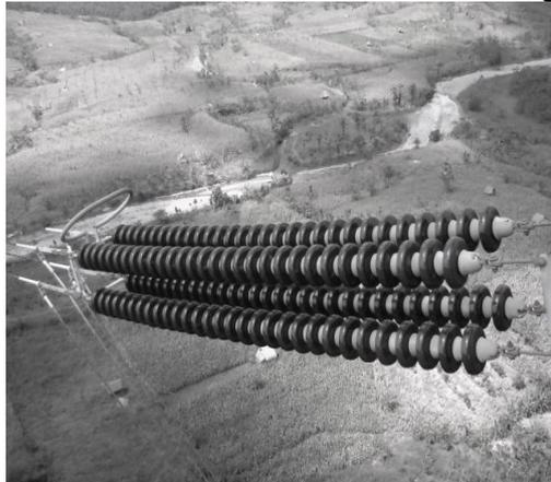
**Gambar 6.20 Insulator *quadruple***
