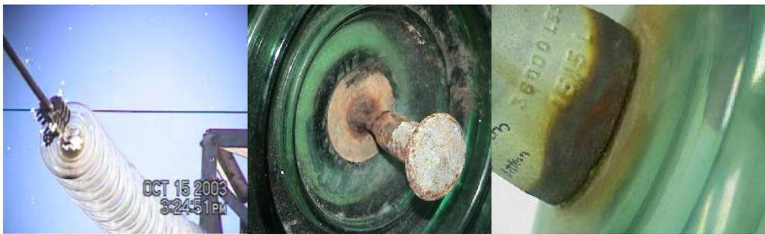
Gambar 6 Korosi Pada Insulator
