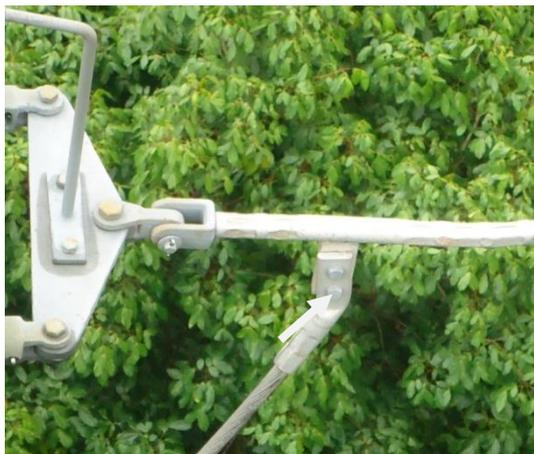
Gambar 6.4 Jumper Joint
