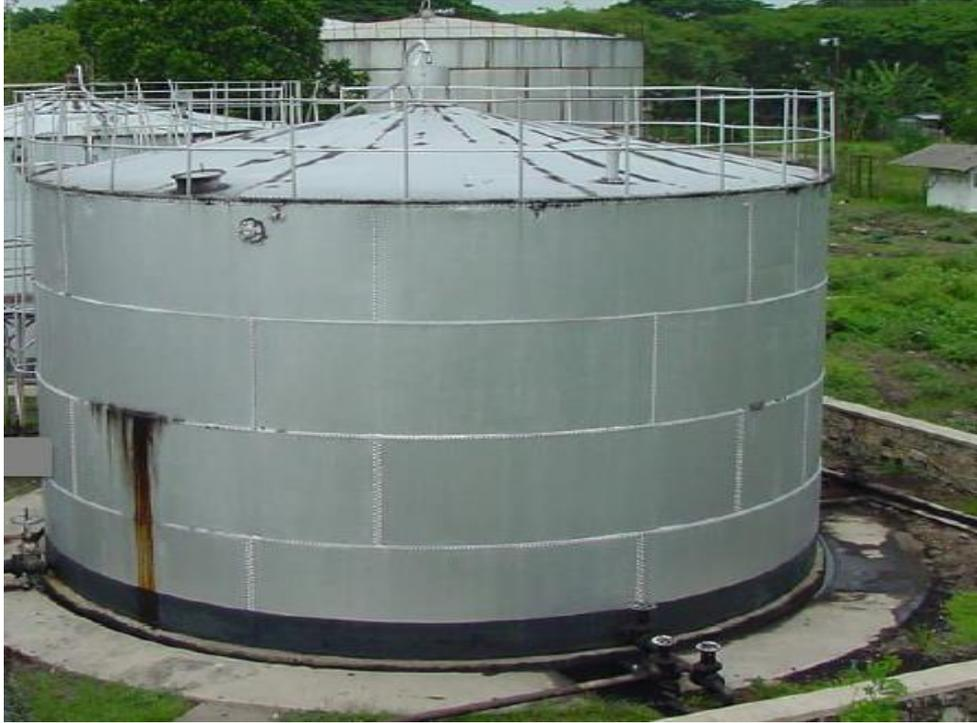
**Gambar 5. Tangki Silindris Tegak Atap Tetap Kerucut (*Fixed Cone Roof*)**
