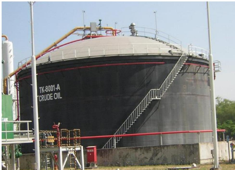
**Gambar 4. Tangki Silindris Tegak Atap Tetap Kubah (*Fixed Dome Roof*)**
