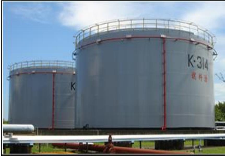
**Gambar 6. Tangki Silindris Tegak Atap Bergerak (*Floating Roof*)**
