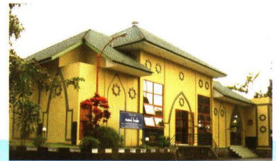
Masjid P4TK-SB Dekat Studio DKV
