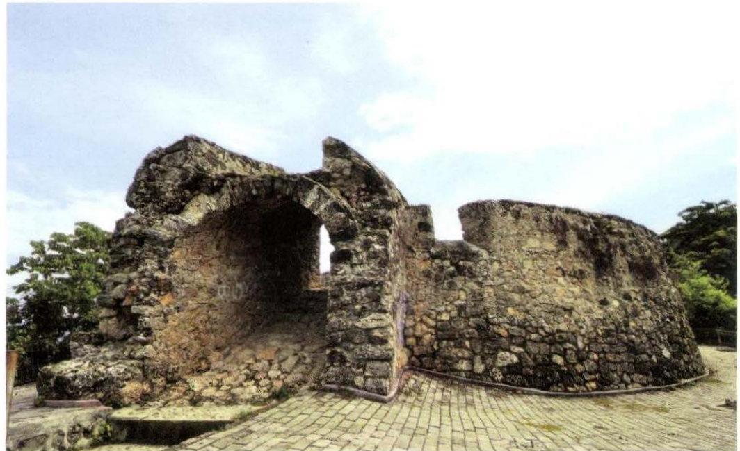
P. 164 The gate built from natural stone forms an arch. Several parts have collapsed.
