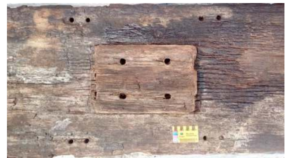
Figure 11. A Lug With Ligature Holes on Each Corner. (Source: A. Mochtar, 18 November 2017)
