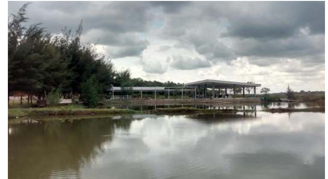
Figure 7. New Shelter of the Boat, During Construction Work. (Source: A. Mochtar, 2 January 2018)
