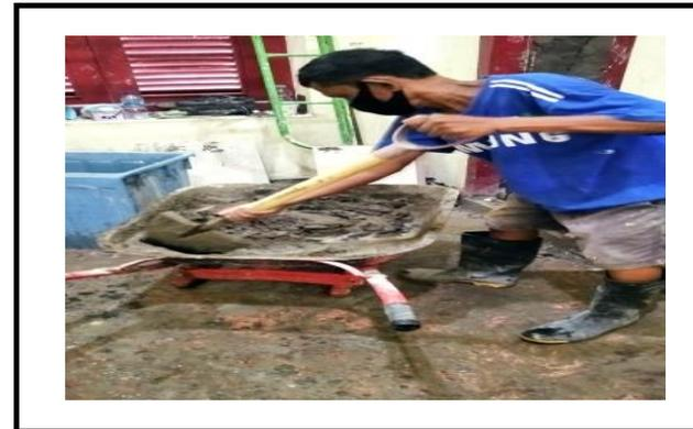
***FOTO KEGIATAN PEMBUATAN ADONAN (CAMPURAN) PEMASANGAN KERAMIK LANTAI DAN DINDING GEDUNG I***
