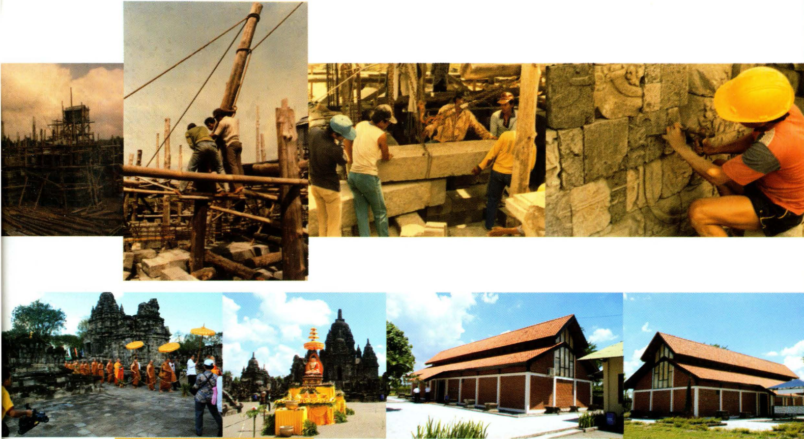
THE RESTORATION OF SEWU TEMPLE Prambanan — Klaten — Central Java
